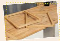
Drill holes into the ends of the boards and connect them to form two identical frames using the screws. Paint the frames if desired.
